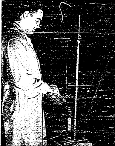
Pouring soil into the mold.
